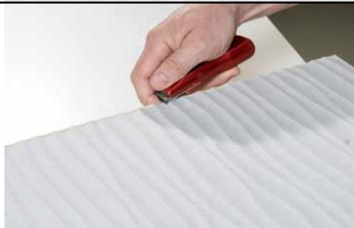
Finally clean surface structure with a sanding pad (approx. grain 100).
